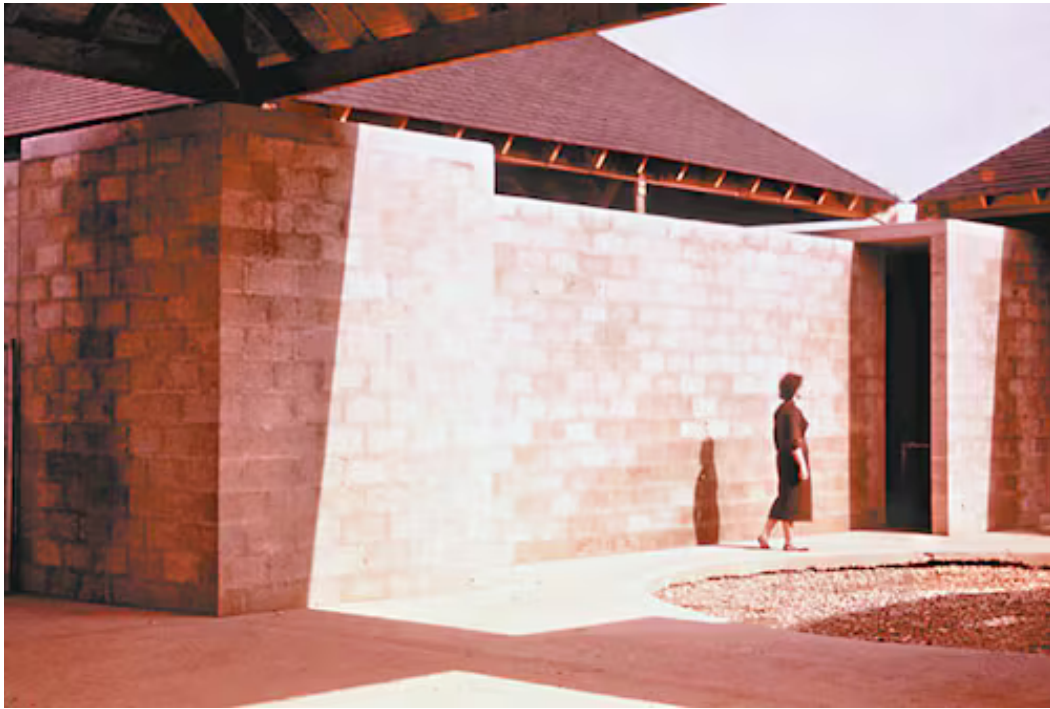
A woman walks through the central court of the Trenton Bath House. (Courtesy of the Architectural Archives, University of Pennsylvania)
