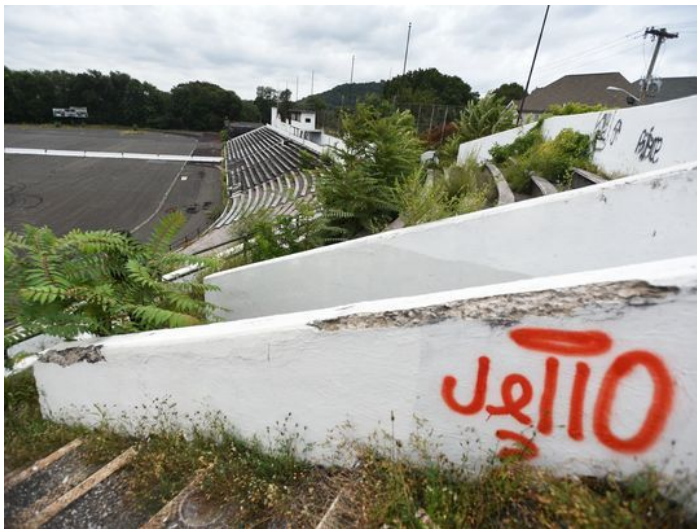
General scene of the historic Hinchliffe Stadium in Paterson on Aug. 29, 2017.
