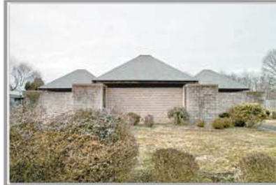
BRIAN ROSE The exterior of Louis Kahn's Trenton Bath House in Ewing Township just before its restoration.
