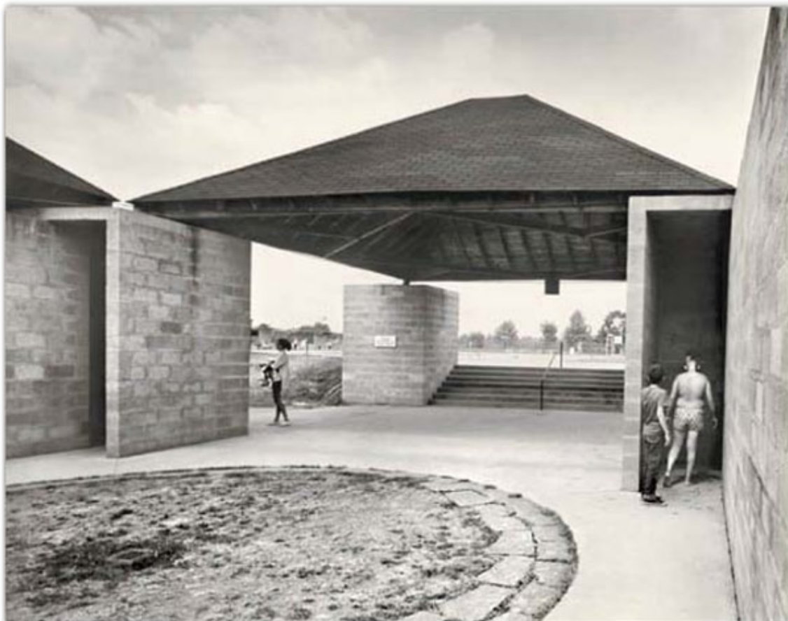
Boys enter the men's changing room through Kahn's baffled entrance of the Trenton Bath House. (Courtesy of the Architectural Archives, University of Pennsylvania)
